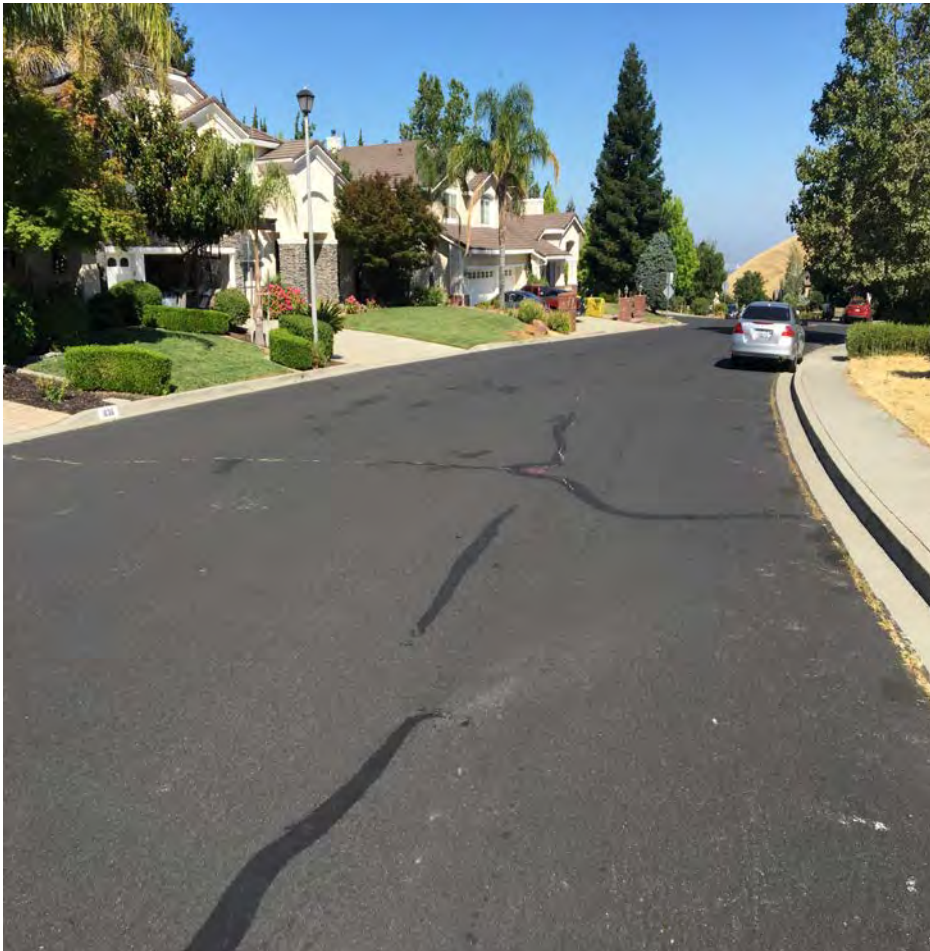
Cracks in AC pavement along Pebble Beach drive in the same location as previous observations. Viewed looking Northwest from the southeast edge of Interpreted deformation zone
